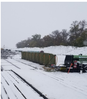
Cleaning station south end of the Michel's HDD site at Dead Horse Creek Photo taken facing South West
