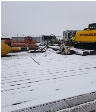
Michel's HDD at Dead Horse Creek Photo taken facing East
