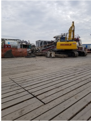
Michel's HDD site at Dead Horse Creek Picture taken South East
