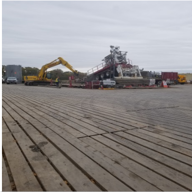
Michel's HDD at Dead Horse Creek Photo taking facing North East
